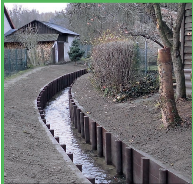
AMX-PL Recycled plastic lumber Retaining wall,, Europe
