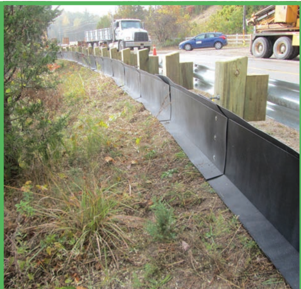
AMX-SP Scored plastic (HDPE) Attached to guardrail, Ontario
