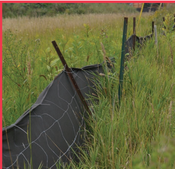
Wire reinforced silt fencing Various species, USA
