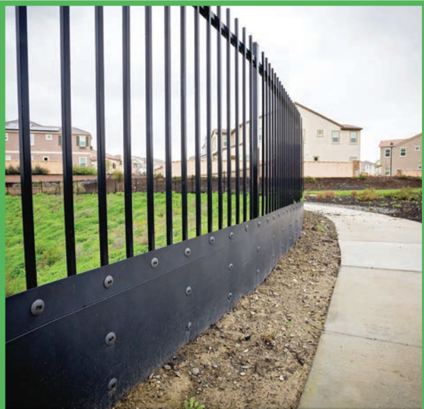
AMX-SP Scored plastic (HDPE) Attached to existing "Garrison" fencing, California
