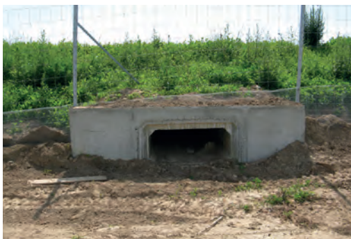
15 Structure head in concrete formwork. Source: Cerema.
