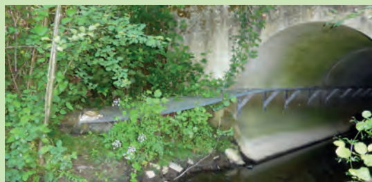
Recycled plastic bench, 50cm wide by 65m long and 70cm headroom. Cost: €15,000 including VAT (2013). RN137 (DIRO). Source: Cerema.
