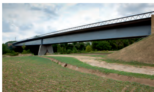
1 Metal structure Source: Matière TP.
