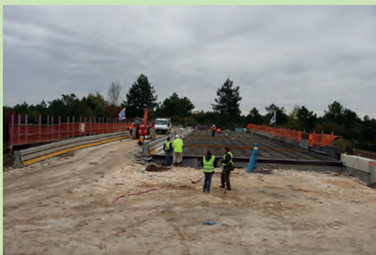
④ Structure under construction. Source: ASF/Vinci Autoroutes.
