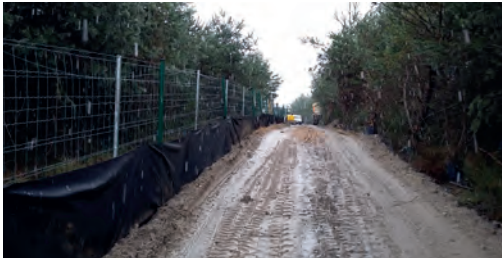
Site access track. Source: ASF/Vinci Autoroutes network.
