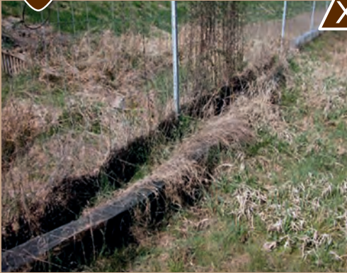
Amphibian fence brought down by the weight of the vegetation. Source: Cerema.
