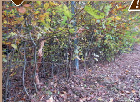
The lack of maintenance of fencing on the outside of the road coverage prevents it from being kept in good condition. Source: Cerema.
