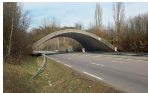
⑤ Arched bridge RD 31, Moselle. Source: Cerema.
