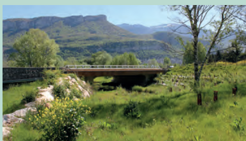
Underpass on the RD121a. Source: Departmental council of Isère.
