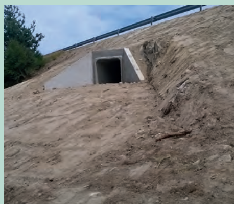
Finalised work before the fencing was installed.
