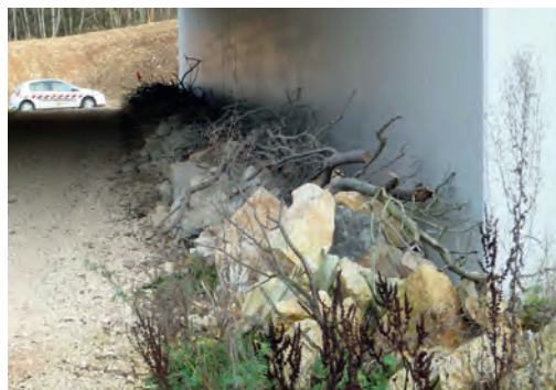
Underpass with swath. RN67 (52). Source: Cerema.
