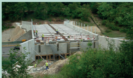
Passage under construction. Source: Vinci Autoroutes/ASF network.
