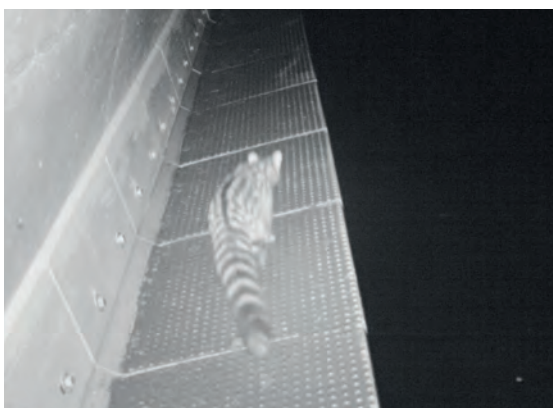
⑥ Genet using a polymer concrete bench. Source: Vinci Autoroutes/ASF network.
