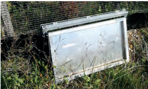
23 Small fauna escape exit in the Netherlands. Source: Cerema.
