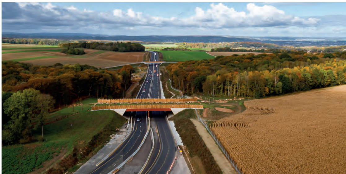
❶ Overpass on the A16 motorway. Source: Sanef.
