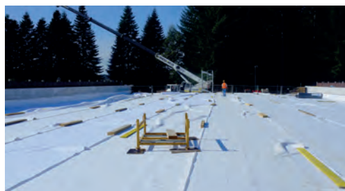
Sealing and drainage phase of the deck. Source: Vinci Autoroutes/ASF network.
