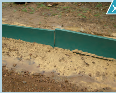
Brittle rigid plastic border, not suitable for road use. Source: Cerema.
