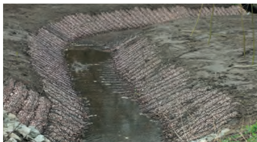
⑪ Reconstruction of banks in gabion mattresses*. Source: AquaTerra Solutions.
