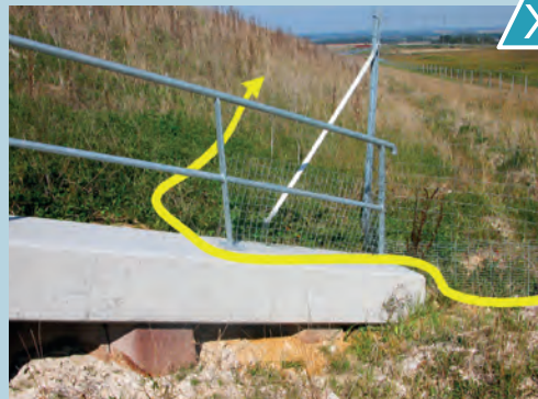
Incorrect connection of the wire fence to the structure allowing wildlife free access to the coverage. Source: Cerema.
