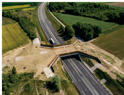
1 Overpass fitted with an abutment on the front wall. Source: ATMB - Arnaud Lesueur.
