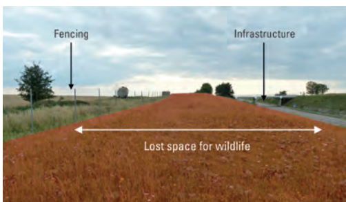
Fencing positioned at the coverage boundary preventing wildlife from accessing green rights-of-way. Source: Cerema.
