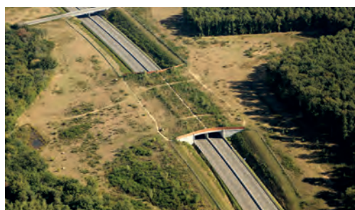
6 Covered trench of the A19 motorway in the crossing of the forest of Montargis. Source: Arcour.
