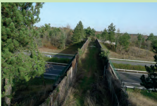
② Initial overpass. Source: ASF/Vinci Autoroutes.
