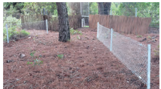
28 Installation of 2 fences guiding towards the device. Source: IMPCF.
