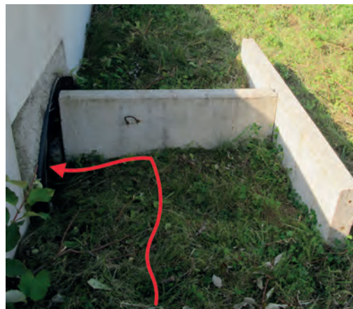
13 Guiding system to facilitate use of the passage by amphibians. Source: Cerema.
