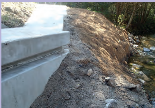
18 Development within the fauna bench of a passageway for micromammals*. Source: P. Fournier GREGE.
