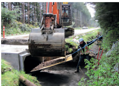
Implementation of a layer of natural materials. Source: Barb BEASLEY, Association of Wetland Stewards for Clayoquot and Barkley Sounds.
