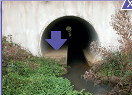
14 Presence of a step at the entrance of the passage limiting access to the smallest species. A34 Reims, Charleville-Mézières. Source: Cerema.
