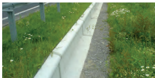
④ Example of a concrete edge. Source: Maibach.
