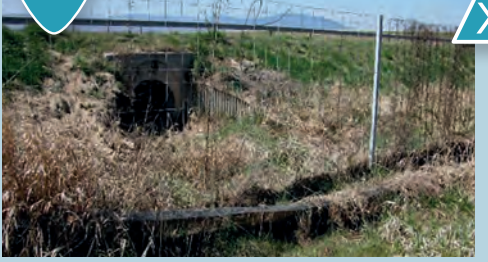
Fencing preventing wildlife from accessing the structure. Source: Cerema.
