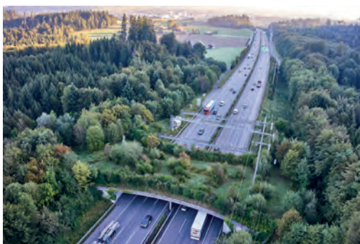
4 Example of a remarkable all fauna passage on the A1 motorway in Switzerland. Source: AURA/Emanuel
