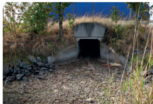
16 Structure head with open walls. Source: Cerema.
