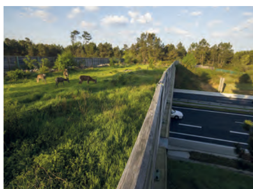
Does on the dedicated overpass of La Lande. A10 motorway. Source: © VINCI Autoroutes photograph library – Emmanuel Rondeau.
