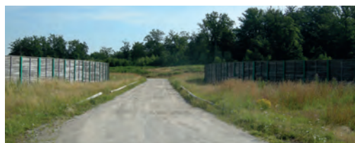
Wooden gates installed along the path to prevent vehicles from accessing the wildlife area. Source: Cerema.
