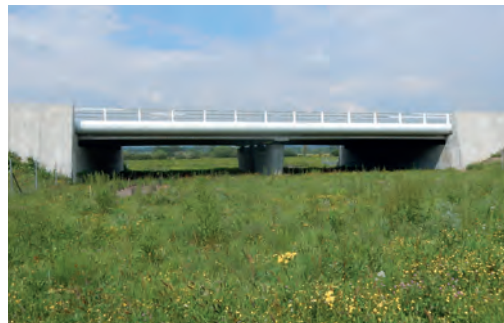
21 Functional hydraulic discharge structure for fauna. A304 motorway (Grand Est region). Source: Cerema.
