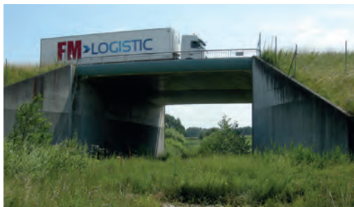
❶ Dedicated ordinary all fauna underpass. RN 4 (54). Source: Cerema.
