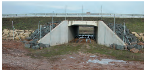
Large fauna fencing bypassing the structure head. Source: Cerema.
