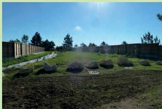
⑤ View of the completed structure. Source: ASF/Vinci Autoroutes.
