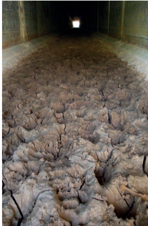
Badger tracks, among others, in a structure of the A35 motorway (Grand Est region). Source: Cerema.
