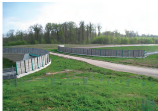
17 Overpass on mixed agricultural/fauna passage. RN 59 (Grand Est region). Source: Cerema.
