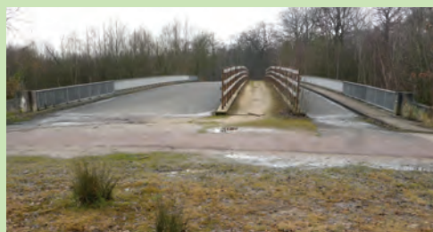
View of the structure before works. Source: Vincent Vignon, OGE.
