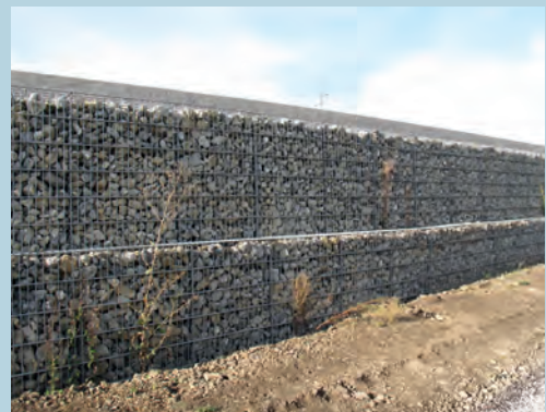
Gabion wall along the RD16 (57). Source: Cerema.
