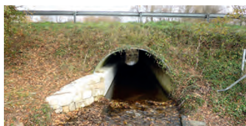
Concrete bench RN 165 (DIRO). Metal duct. Source: Cerema.
