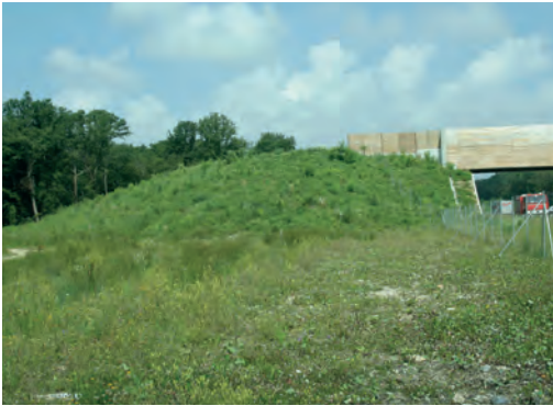
③ Access ramp to the fauna passage. RD64 (70). Source: Cerema.
