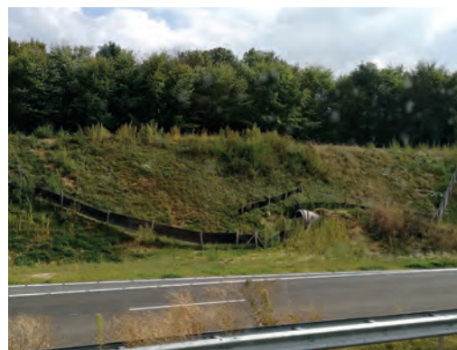
8 Example of a small fauna passage with a sloping structure head parallel to the infrastructure. Source: Cerema.
