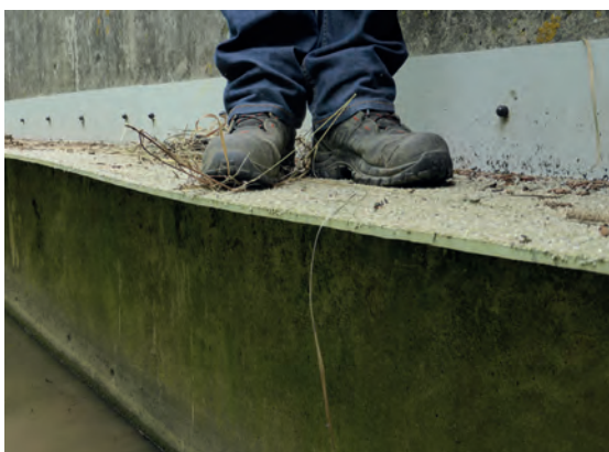
④ ⑤ GRP bench, 50cm wide by 67m long and with 200cm headroom. Cost: €35,000 including VAT (2015). A83 motorway. Source: Cerema.
