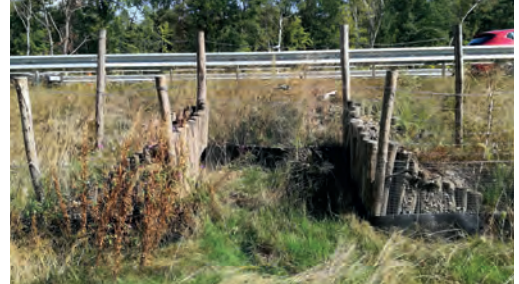
Escape exit with double ramp (Netherlands). Source: Cerema.
