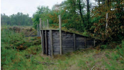
Escape exit with a single ramp system (Netherlands). Source: Vinci Autoroutes.
