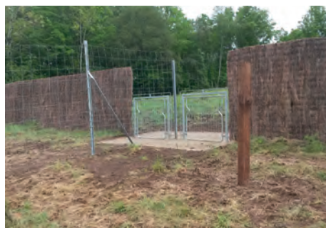
Hatch accompanied by a guiding fence. Source: Vinci Autoroutes/ASF network.
