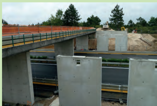
③ View of the piers. Source: ASF/Vinci Autoroutes.
