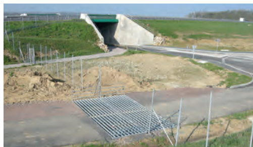
15 Cattle grid installed to prevent wildlife from accessing the infrastructure from a secondary road. Source: Cerema.
