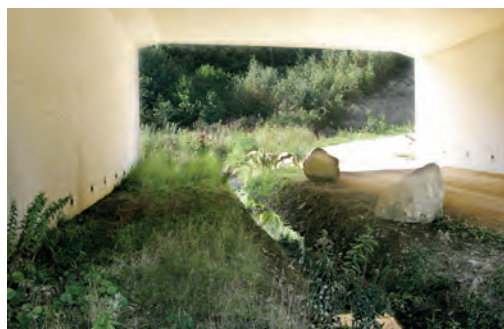
Underpass in which uses are separated by blocks and the passage of a watercourse (A34 motorway). Source: Cerema.
