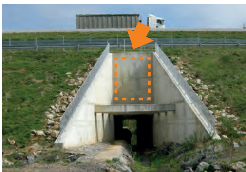
24 Olzey stream structure. RN 59 (54). Source: Cerema.
