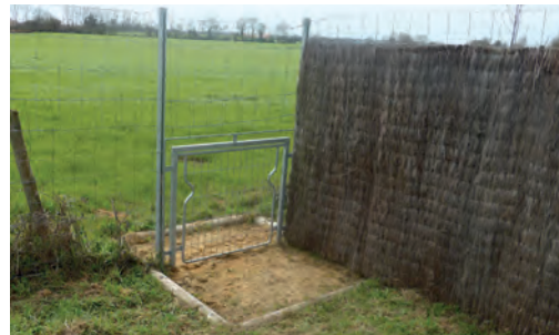
22 Escape exit, Vinci Autoroutes network. Source: Cerema.
