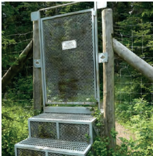
6 Gate equipped with access steps to reduce the possibilities for wildlife to enter. Source: A. Clevenger.
