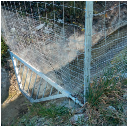
12 Example of devices put in place to ensure the continuity of fencing: removable grid on ditch. Source: Cerema.
