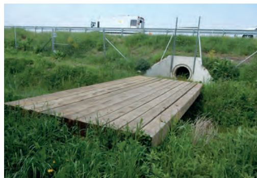
⑫ Wooden platform used to cross a ditch. Source: Cerema.
