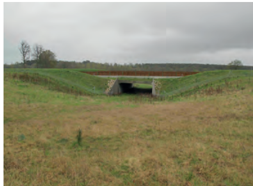
8 Underpass with funnel pit. A88 motorway (Orne). Source: Cerema.
