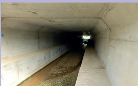
Frame element equipped with a prefabricated concrete bench. Source: Cerema.
