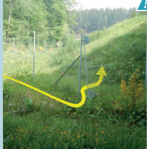
Opening in the fencing allowing access to the coverage. Source: Cerema.
