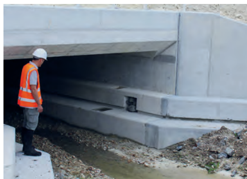
17 Example of shelters created in the fauna bench of a structure. Source: Michel Bramard OFB.
