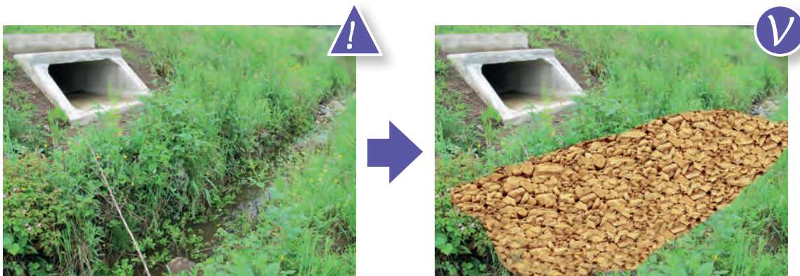
14 Schematic example of a ditch crossing system by filling with draining materials. Source: Cerema.
