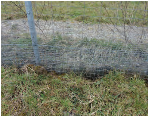
Example of a fine-mesh fence backed by a large fauna fence with progressive meshes. LGV Est. Source: Cerema.
