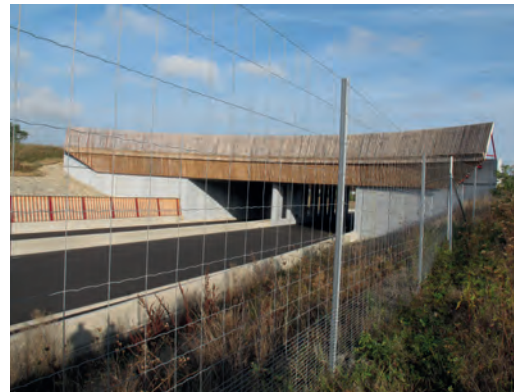
Example of a large fauna fence with progressive meshes. RD 16 (CD57). Source: Cerema.
