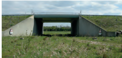
22 Underpass of equivalent height to the embankment. RN 4 (54). Source: Cerema.
