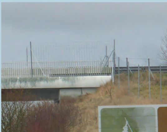
Return on civil-engineering structure. Source: Cerema.
