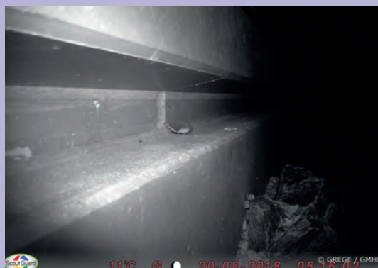
18 Development within the fauna bench of a passageway for micromammals*. Source: P. Fournier GREGE.
