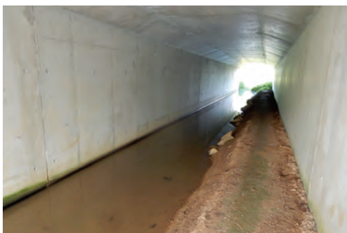
Example of a bench made in natural materials. Source: Cerema.
