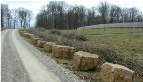
17 Stone blocks positioned along a forest restoration of the LGV Est Européen high speed train line. Source: Cerema.
