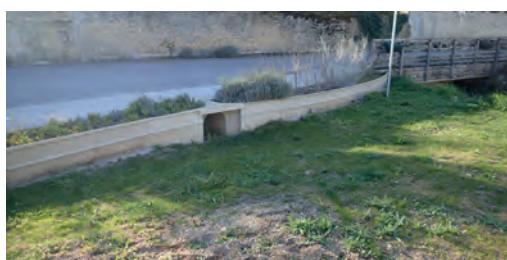
2 Polymer concrete edge. Source: Environment committee, municipality of Ahuy.
