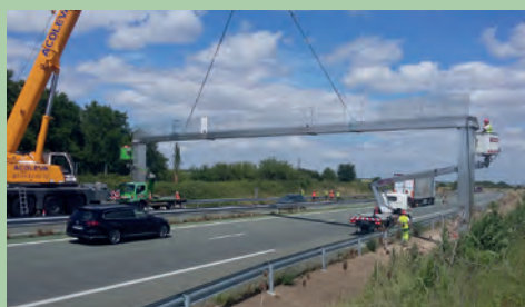
Installation of the gantry. Source: Vinci Autoroutes/ASF network.
