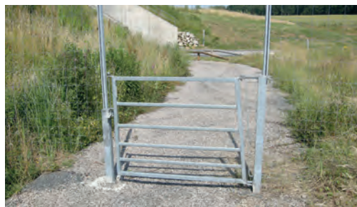
16 Pedestrian gate whose hinges are offset (closer to the post at the bottom than at the top) so that it closes automatically without intervention. Source: Cerema.
