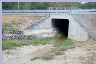
Stepped bench (concrete). Source: P. Fournier GREGE.
