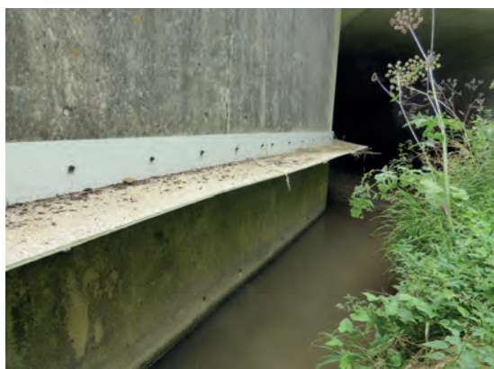
④ ⑤ GRP bench, 50cm wide by 67m long and with 200cm headroom. Cost: €35,000 including VAT (2015). A83 motorway. Source: Cerema.
