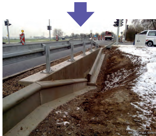
Structure equipped with an access ramp. Source: Maibach.
