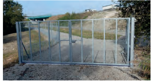
4 Gate equipped with a "skirt". Source: Cerema.
