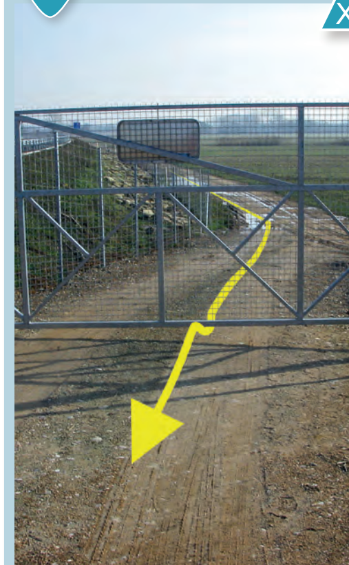
Space available under the gate allowing small fauna to pass. Source: Cerema.
