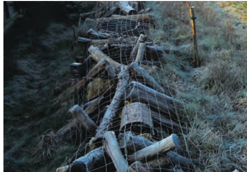
12 Fenced swath to avoid theft and the disposal of objects on the motorway. Source: Vinci Autoroutes.
