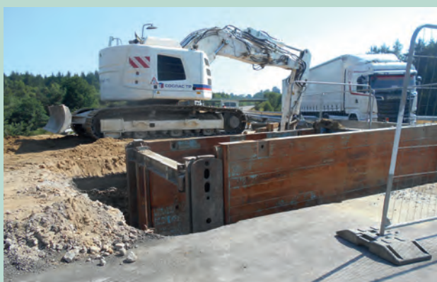
Opening of the roadway and reinforcement of the trench.
