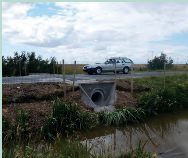
Finalised structure with fence device to prevent the otters from returning to the roadway. Source: François Varenne.
