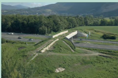
La Buisse passage on the A48 motorway. Source: R. Courtaud - AREA.
