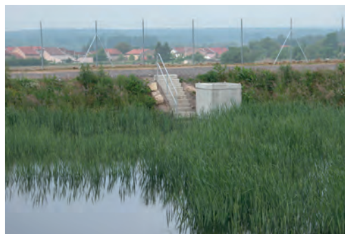
⑳ Retention pond equipped with amphibian fences. Source: Cerema.
