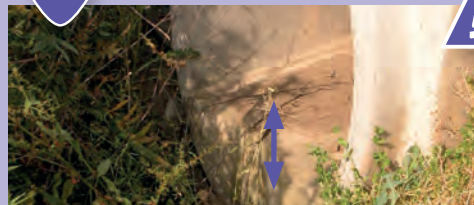
17 Presence of a step at the entrance of the passage preventing access to smaller animals. Source: Cerema.
