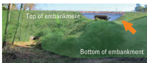
Underpass positioned at the top of the embankment. Source: Cerema.
