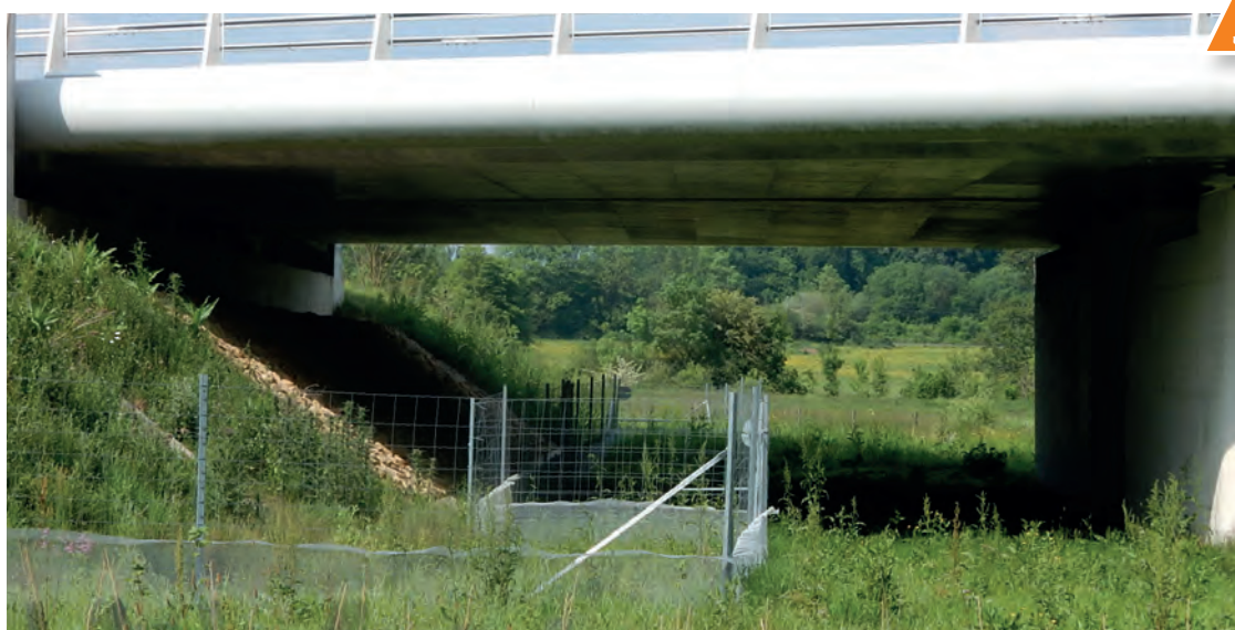
Fencing that hinders the movement of wildlife. Source: Cerema.
