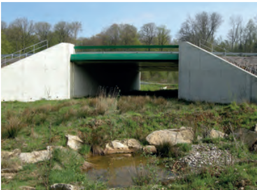
7 Underpass on the RN 4. Grand Est region. Source: Cerema.
