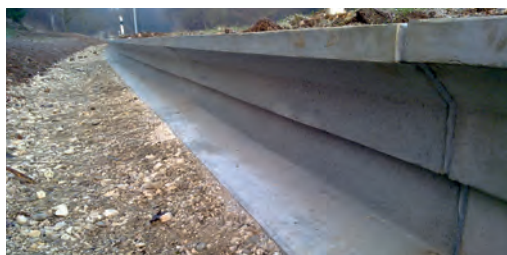
1 Concrete edge Source: Maibach.
