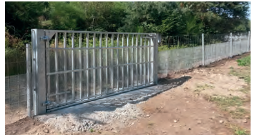
5 Gate equipped with a concrete threshold. Source: Vinci Autoroutes/ASF network.
