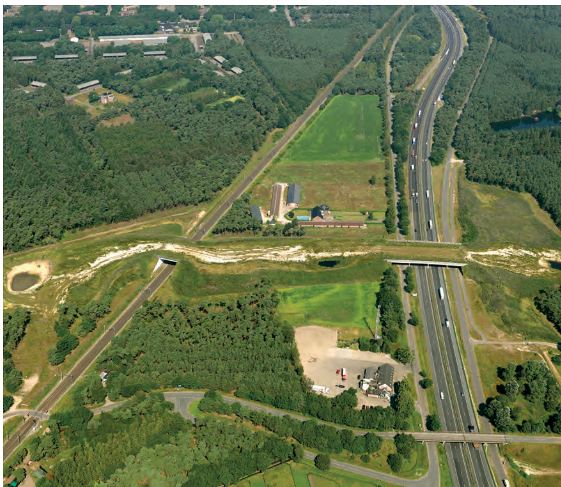
☺ All fauna passage equipped with a pond at each entrance of the passage. A2 motorway north of Eindhoven. Source: Luchtfoto Irvin Van Hemert – Netherlands.
