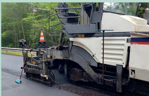
Surface repair. Source: Cerema.
