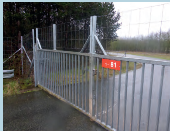
Height extension on service gate. Source: Cerema.
