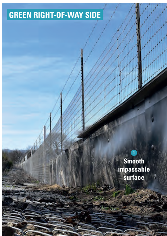
High density polyethylene barrier attached to a fence. Source: Animex Fencing.
