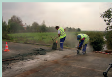
Opening of the roadway for laying the elements of the structure. Source: François Varenne.
