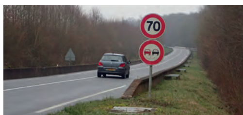
15 Concrete wall guiding amphibians and securing users. Source: Cerema.
