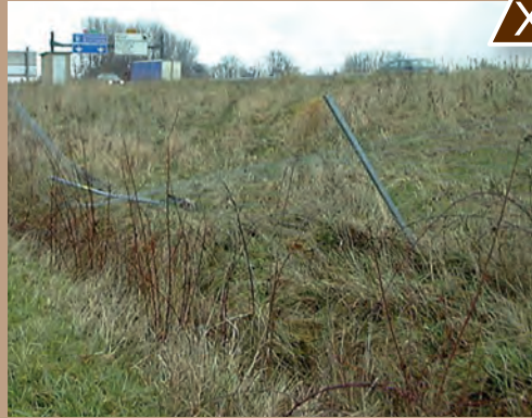
Fence damaged during a traffic accident. Source: Cerema.
