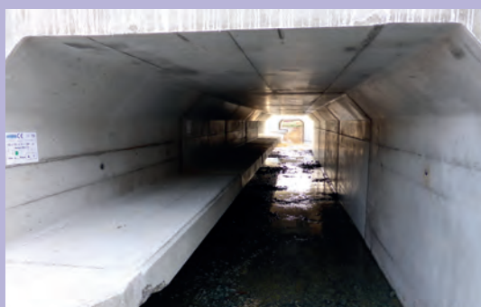
Frame element equipped with prefabricated concrete corbelling. Source: Cerema.
