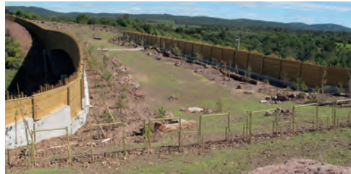
18 Chicane system installed on the A57 motorway overpass. Source: Jean Carsignol.
