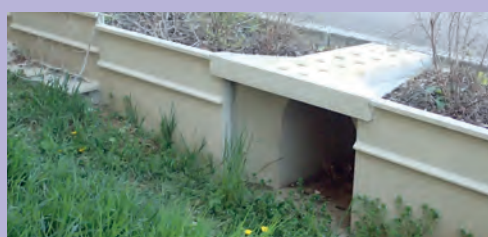
Open-worked crossing structure. Source: Environment committee, municipality of Ahuy.
