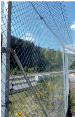
Example of a fence with a flap for lynx. B10 motorway, Germany. Source: Cerema.
