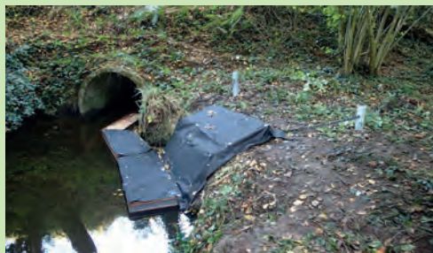
Connection of the Pontoon to the bank. Source: GREGE.
