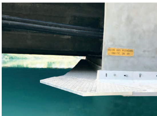
⑦ Polymer concrete bench with non-slip device. Source: ULMA Architectural Solutions.
