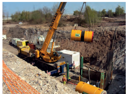
Setting up of microtunneling on a railway track. Source: Christian Chéreau - SNCF Réseau.
