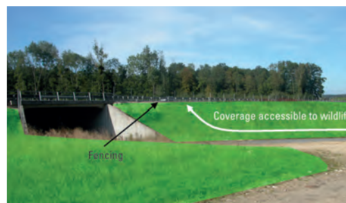
Fencing positioned as close as possible to the road and allowing free access of wildlife to green rights-of-way. Source: Cerema.
