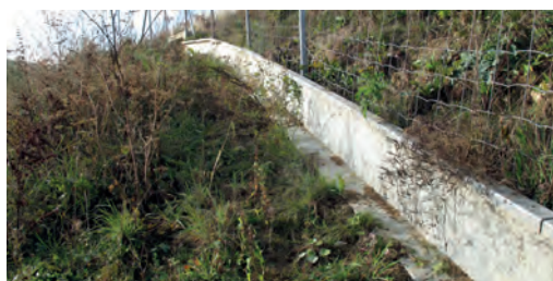
3 Metal edge crowned by a fauna fence. RD16 (CD57). Source: Cerema.
