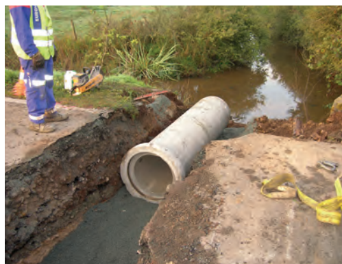
Installation of dry ducts dedicated to otters. Source: François Varenne.
