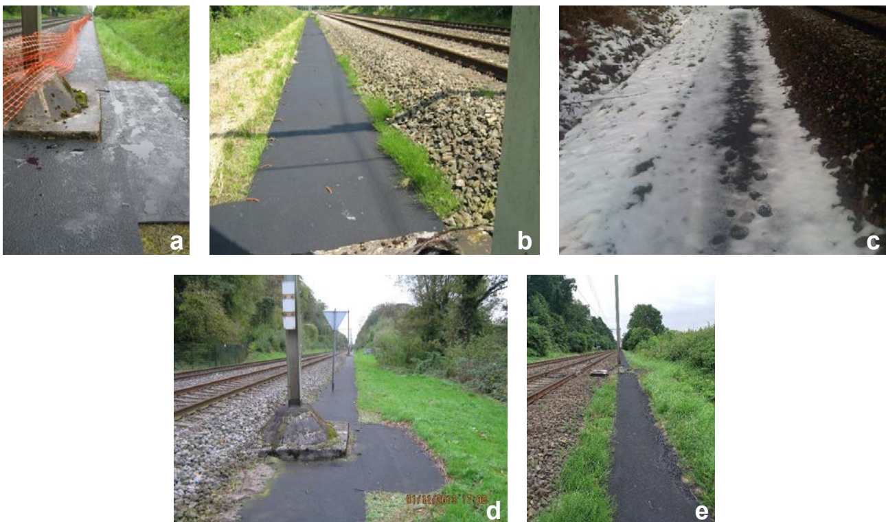
Figure 12: Anti-vegetation mats - ProRail (a) October 2009, (b) June 2010, (c) December 2010, (d) November 2013, (e) July 2019
