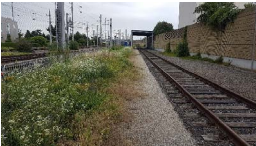
Figure 54: 4-ÖBB-Infra root barrier status after 2 years University of Applied Sciences Carinthia
