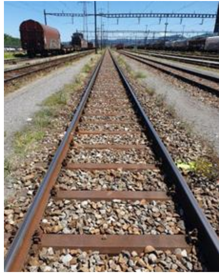
Figure 23: SBB Hot water case study - Reference track, not treated
