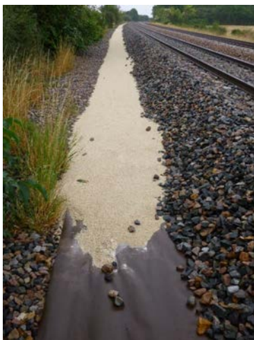
Figure 50: Geotextile laying and covering
