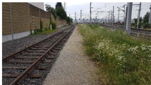
Figure 56: ÖBB-Infra Root barrier status after 2 years University of Applied Sciences Carinthia
