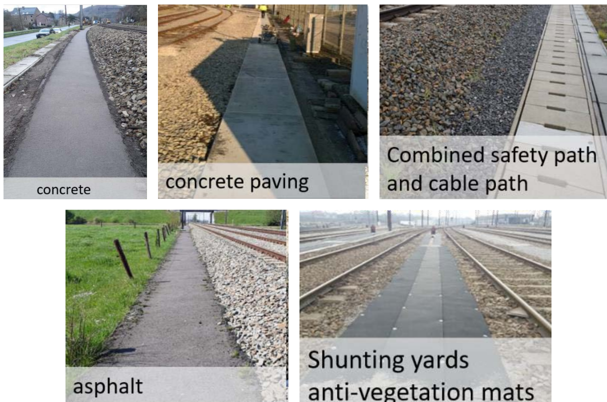
Figure 70: Infrabel - Preventive methods- materials for walkways
