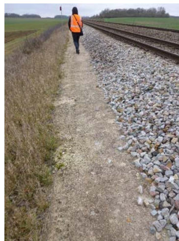
Figure 51: Geotextile laying and covering after 5 years
