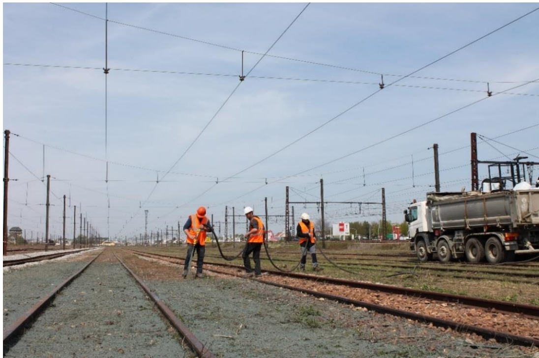
Figure 15: SNCF- Hydroseeding works on service tracks
