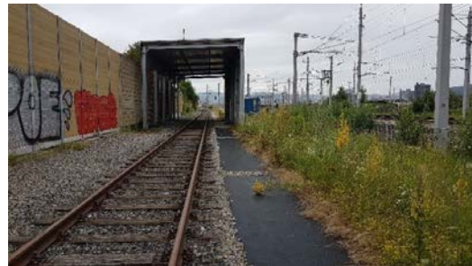
Figure 55: ÖBB-Infra rubber mats status after 2 years University of Applied Sciences Carinthia
