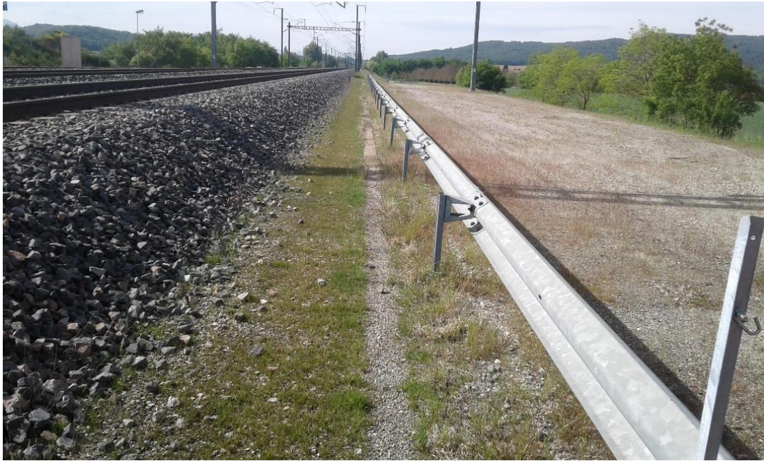
Figure 14: SNCF- Seeding on walkway of high-speed line
